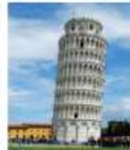
Leaning Tower of Pisa, Italy
