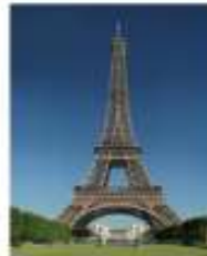
Eiffel Tower, France
